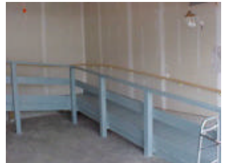
Ramp inside garage
