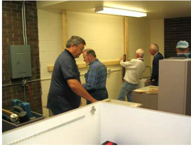
Installing cabinets in the Student Council Store
