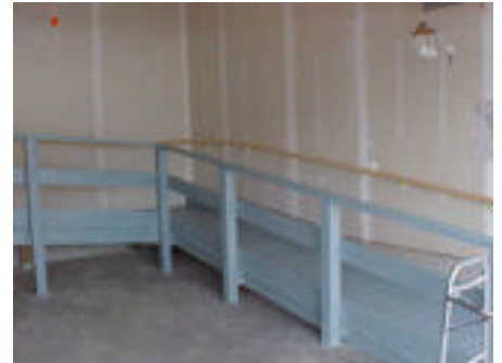
Ramp inside garage
