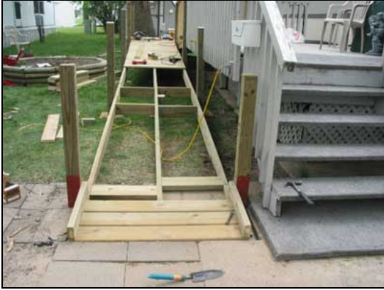
Figure 12. Ramp frame. Notice cross braces.
