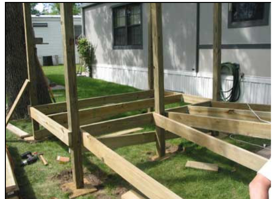
Figure 9. Ramp frame with 180° landing. Notice cross bracing
