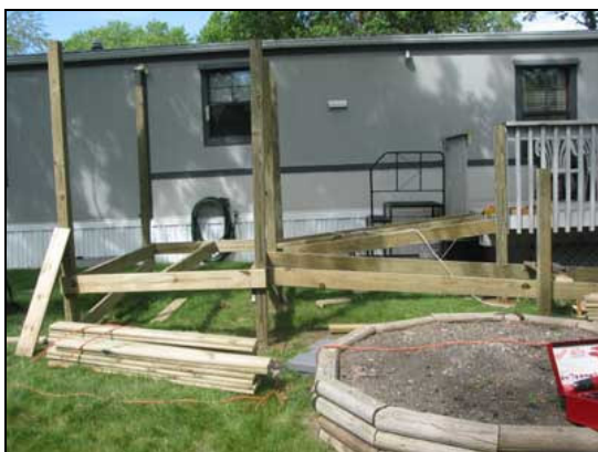
Figure 10. Ramp frame
